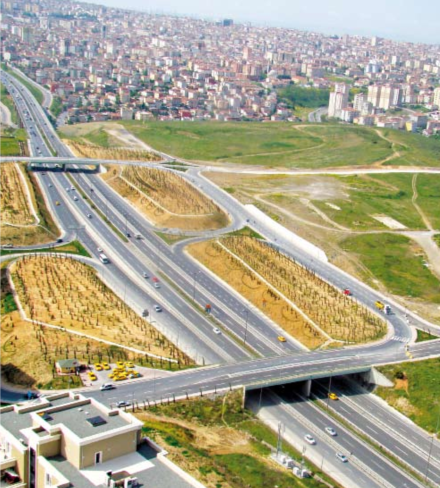
İstanbul-Ataşehir Köprülü Kavşak
